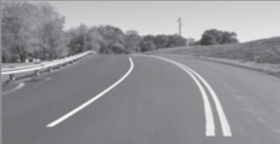
Allison Hollow Road Improvements Chartiers Township
